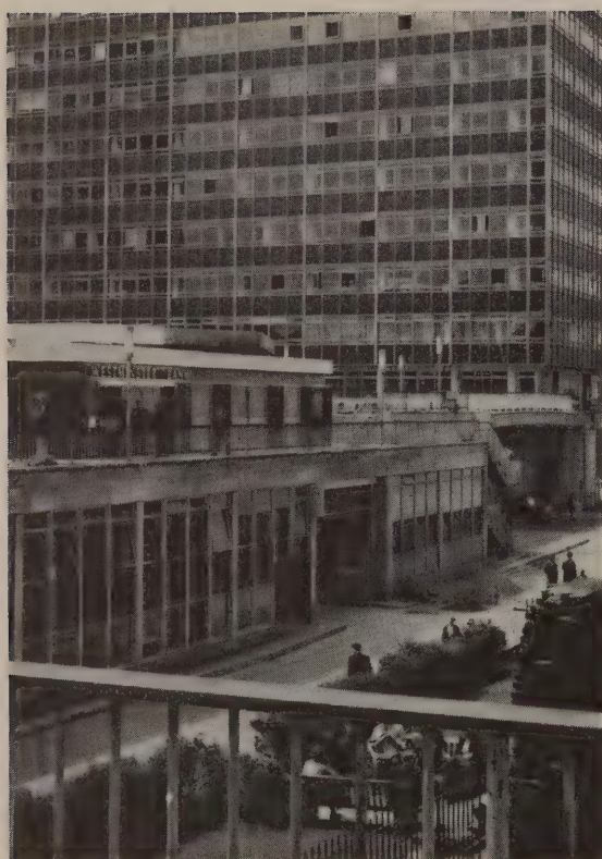
217 The Barbican redevelopment in the City of London. Still under construction, but the photograph shows clearly the beginning of the upper level pedestrian system.
